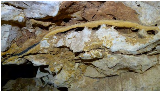
Figure 210: A layer of soft material in solution-modified rock. Photo Darren Brooks
