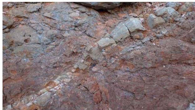
Figure 109: The bedding layer in the entrance of Saddle Cave. Photo Darren Brooks
